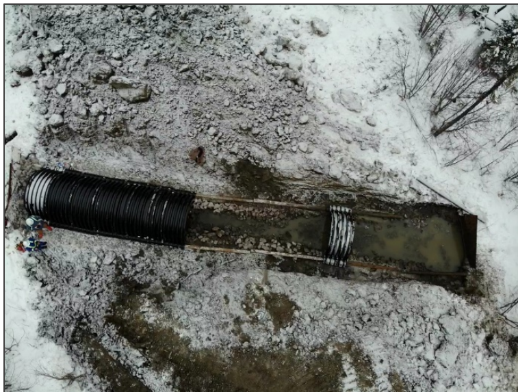
Figure 4. Overhead view of a watercourse crossing reconstruction.
