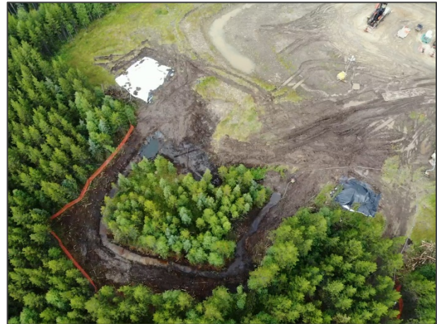
Figure 1. Overhead view of spill pathway at remote pipeline release site.
