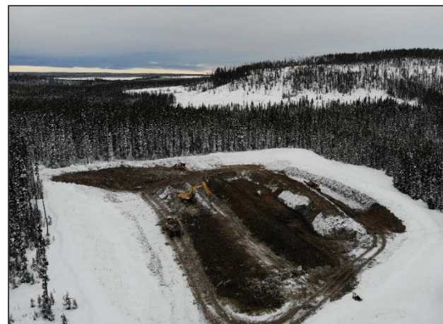
Figure 3. Overhead view of treated soil removal at a remote impacted soil phytoremediation site.
